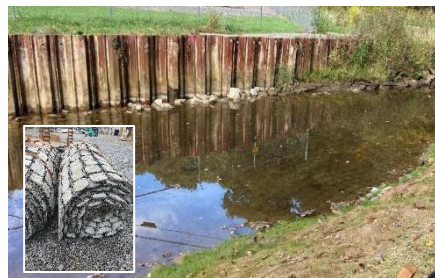
Stabilized bed with cutting-edge materials, after.
