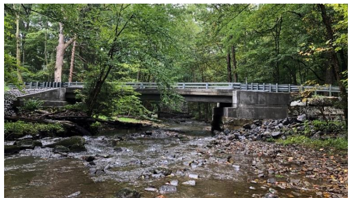
Dotter Road Bridge, before (Left) and after (Right). Photo Credit: Travis Lees, STV
